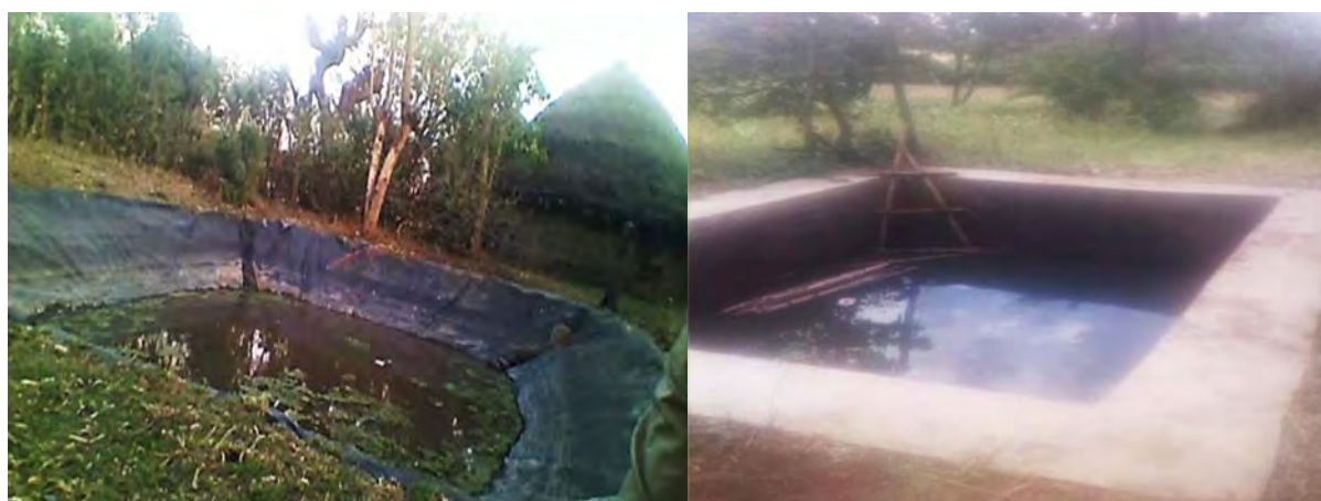
Fig. 1 Left: Plastic lined, and Right: Cement lined HH ponds in Dalocha district, CRV (Photo by the Author, 2019).
